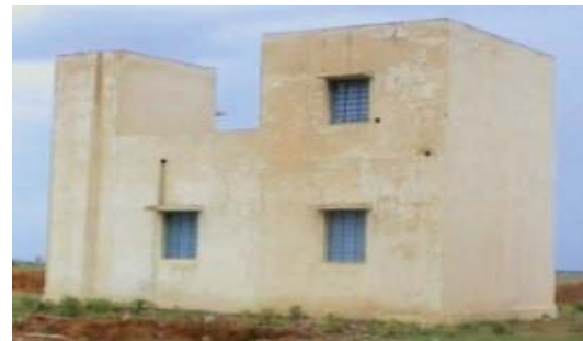
Photograph 3: Double storey three room RCC structure at Sonapur Bazari Project.
