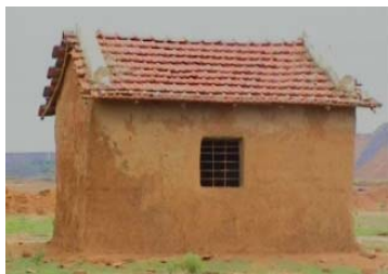
Photograph 1: Single room mud house with Raniganj tiles at Sonapur Bazari Project.
