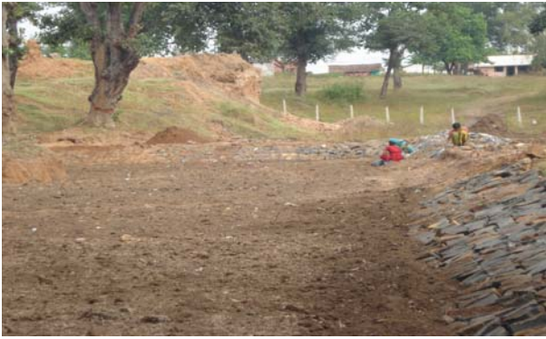
Figure 4: Wetland bed under preparation
