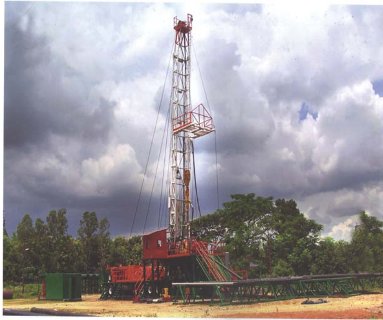
Fig 2: CBM Rig Unit deployed at Moonidih
