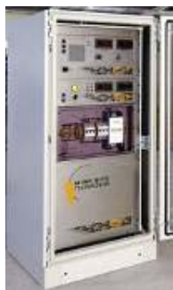
Figure 9 :TTE PAGING ULF transmission headend
