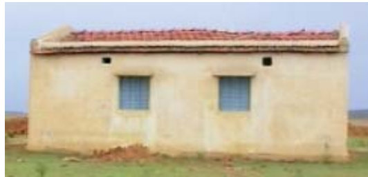
Photograph 2: Single storey two room unit of brick and mud with cement plaster and Raniganj tiles at Sonapur Bazari Project.
